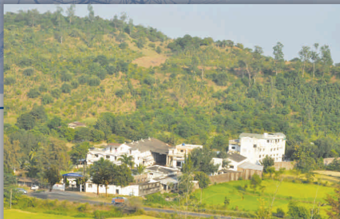
HEX - BCA factory at Vapi, Gujarat
